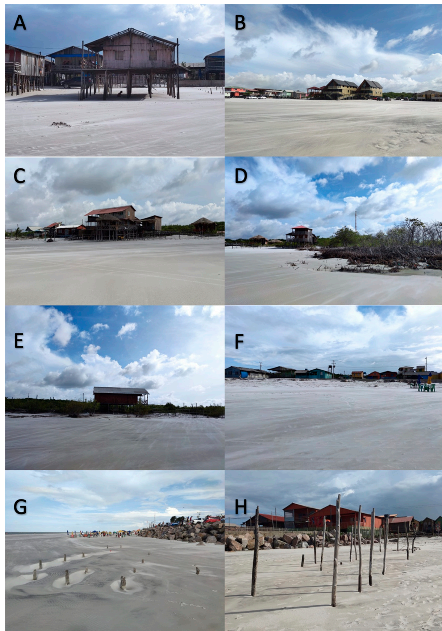
Figure 9. Representation of unregulated development across various areas: intertidal beach zones (A–C), frontal dunes (D–F), and debris from houses located in front of seawalls (G,H).
